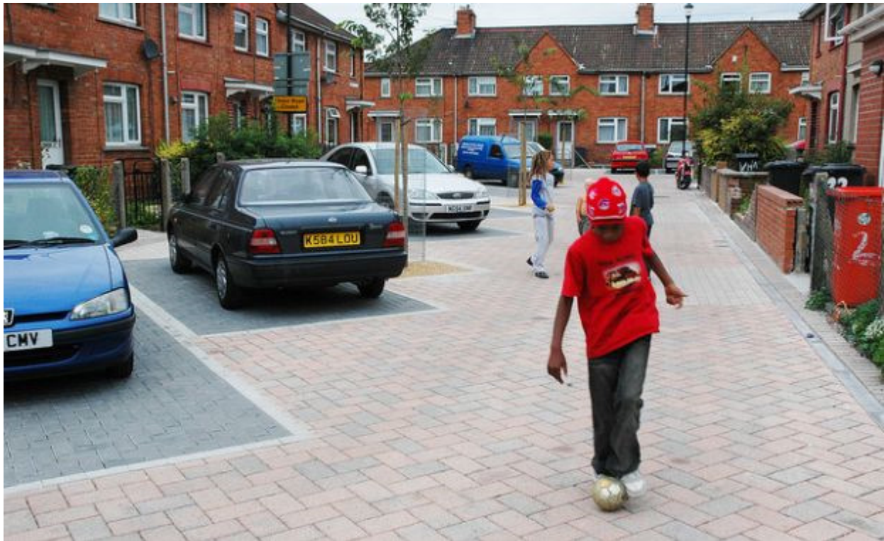
Figure 8: example of homezone shared surface street which uses paving materials combined with embedded kerbs to encourage a low-speed shared environment
